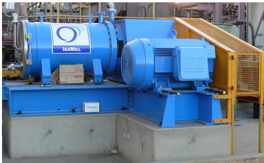
Figure 11: M500 IsaMill™ with 200 kW motor at Cosmos Concentrator
