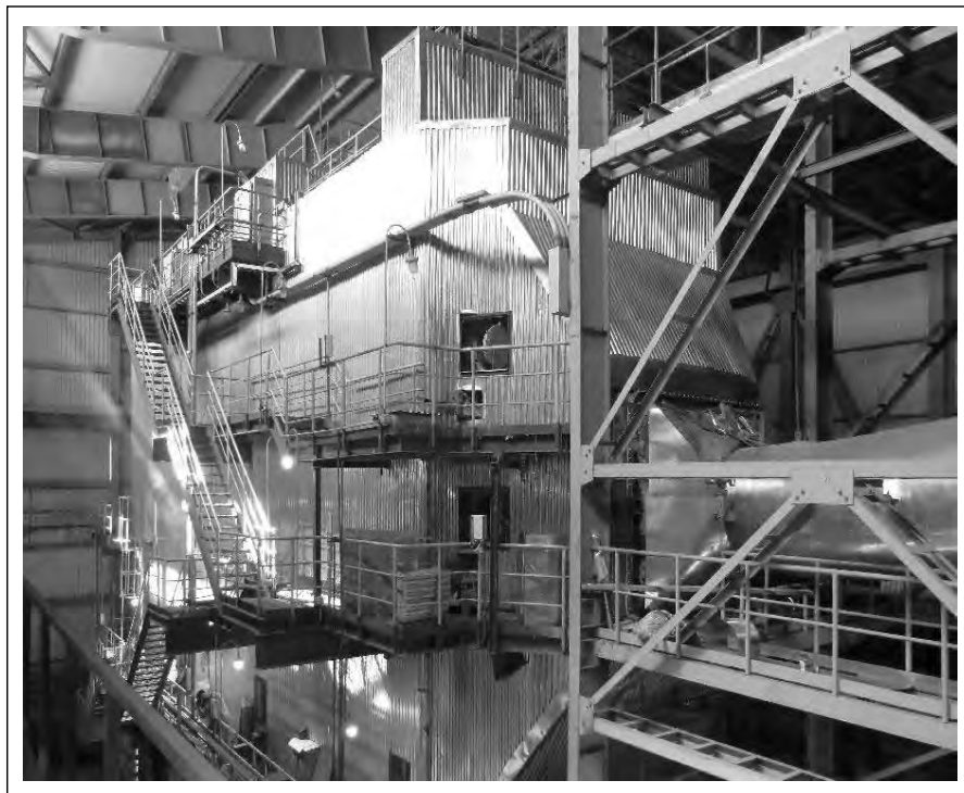
Figure 4: ESP in the Lead plant
