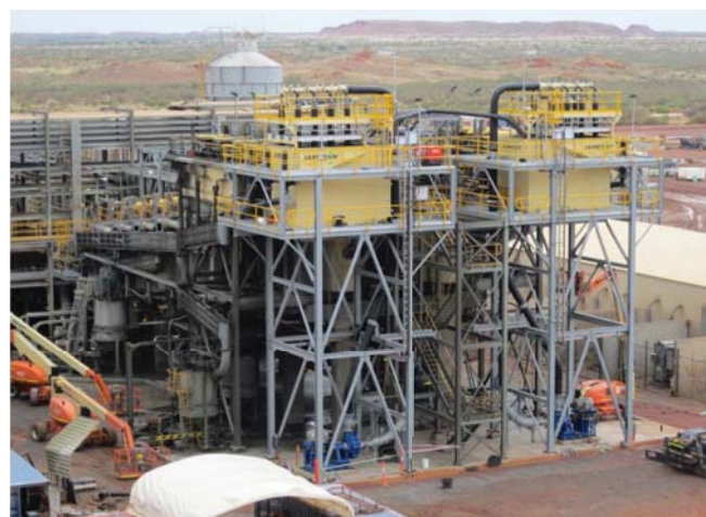
FIG 4 - Photograph showing the installation of the Jameson (cleaner-scalpler) flotation cells at Telfer.
